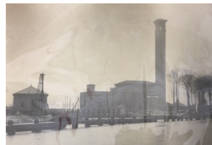
Fig 2.2 The East London Waterworks
