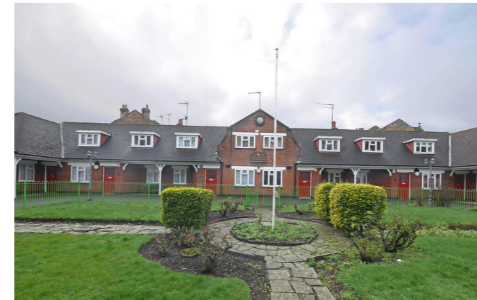
Fig 4.3 Front view of former Disabled Sailors & Soldiers Home, Wattisfield Road
